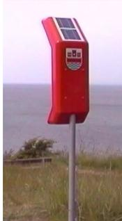
**Figure 2 (left).** PV powered emergency phones at North coast of Sealand (Copenhagen Telephone Company, built 1997).
