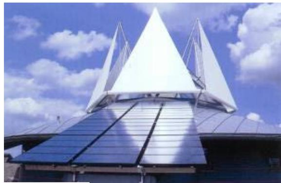
**Figure 1 (above).** Villa Vision at the Danish Technological Institute, Tåstrup (built 1993, with both 2.3 kW m-Si PV modules and also thermal panels).
