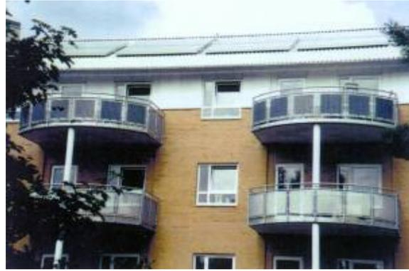
**Figure 9 (above).** Balcony PV retrofits in Herning (2kW c-Si, installed 1997).
